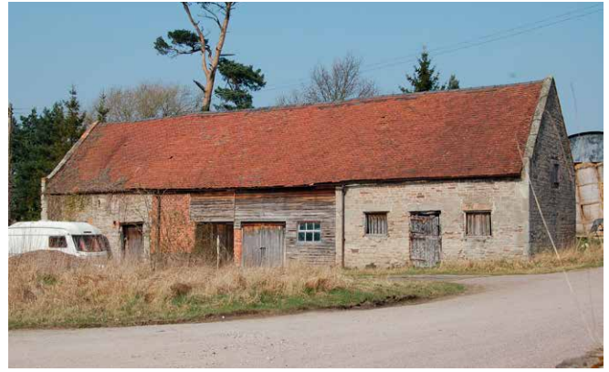
Figure 10 Multi-functional agricultural building, Morville, Shropshire. This unlisted structure illustrates how historic agricultural buildings see adaptation and change over the centuries. Even so, they tend to remain legible. Here it is immediately obvious the right-hand end, with a broad central door and generous flanking windows, was built as a stable. But internal inspection would be needed to see if its fittings survive; it is these which most lend stables their special interest.
