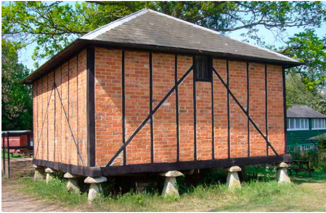
Figure 7 Granary, Pike's Farm, Haversham, Buckinghamshire (now at Chiltern Open-Air Museum, Chalfont St Giles, Buckinghamshire). Granaries, used to store heavy sacks of grain, are necessarily robust buildings; that, coupled with their elevation off the ground which reduces rot, means they tend to survive relatively well. Even late examples, such as this of about 1840, tend to be firmly in local vernacular traditions.
